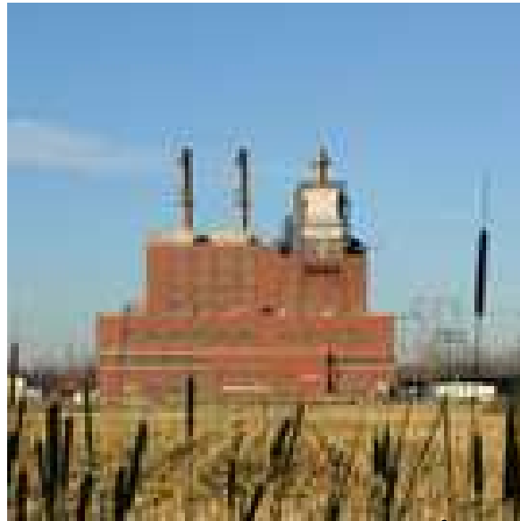
Figure 2 – Existing Sutherland plant 2
